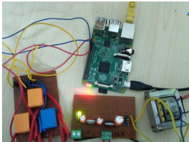
Fig:- Relays connected to the Microcontroller
