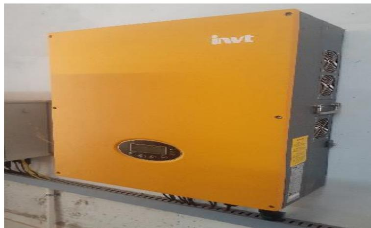
**Fig.3. Solar grid inverter**
